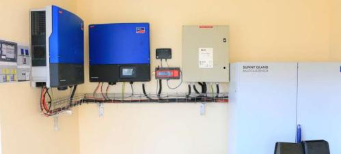
TECHNICAL SPECIFICATIONS PV inverter: Sunny TriPower STP 15000TL-30 Battery Inverter: 2x Sunny Island SI 8.0 H Nominal Battery Capacity: 1940 Ah Communication: Sunny Home Manager 2.0 SMA Cluster Controller
